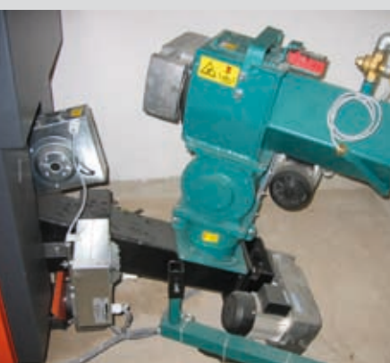
4 chamber rotary valve with counter blade.
