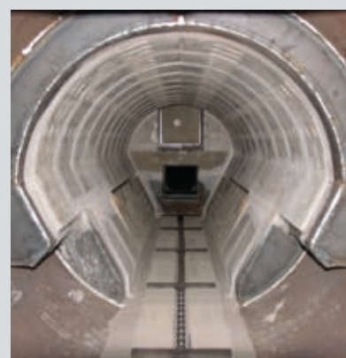
Combustion chamber with de-ashing chain.
