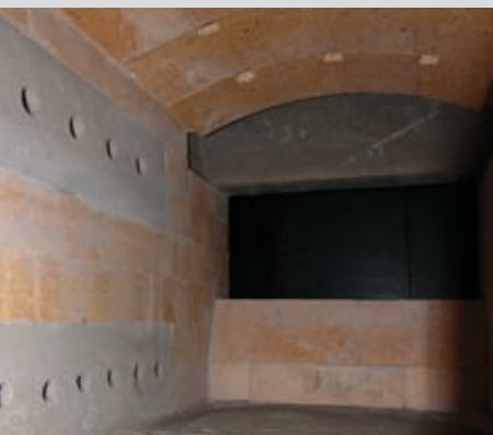
Fully fireclay lined combustion chamber.
