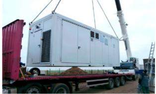
b) Wood gasifier + engine pre-assembled for integration into existing buildings
